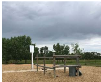
Fox Lake Campground provides a very basic common dumping station for RVs and trailers.
