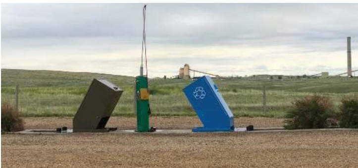
Prairie Oasis Campground provides a robust common dump station with water services to wash the septic tanks after dumping.
